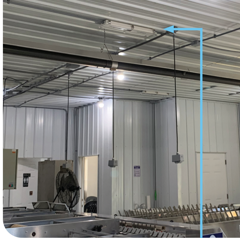
One of thirteen Apex Far-UVC fixtures installed to continuously inactivate pathogens throughout the production area.
